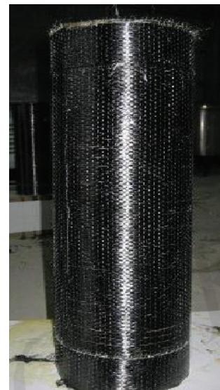
Fig. 1 – Fibre cloth covered reinforced concrete column
